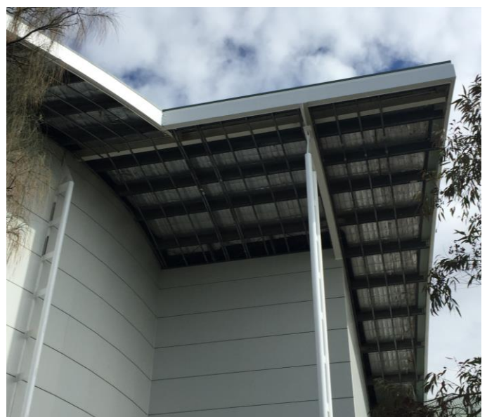
Damaged Sheet Removed
