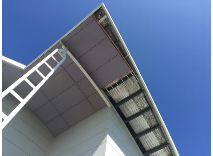
16mm MULTIPANEL INSTALLED on battens at 450mm centres
