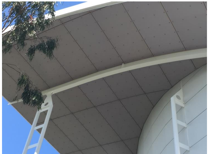
16mm MULTIPANEL installed, ready to be painted
