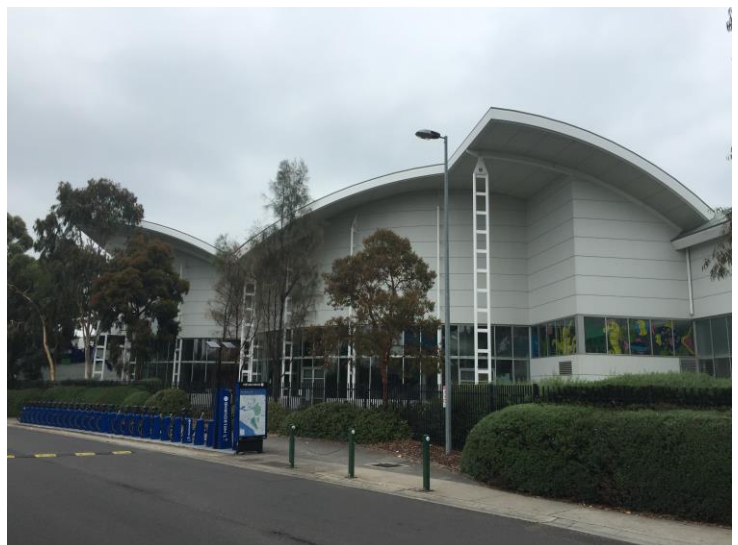
Finished MULTIPANEL installation at MSAC
